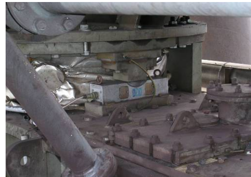
Latest Concept since 2003 - Loading beams Improved weighing accuracy.
