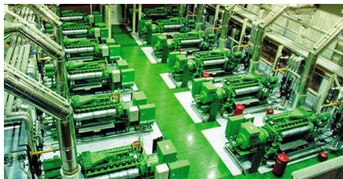
Figura 2: Usina com gás de coque "Profusa SA"; 12 x J316GS; 7.16 Mwe.
