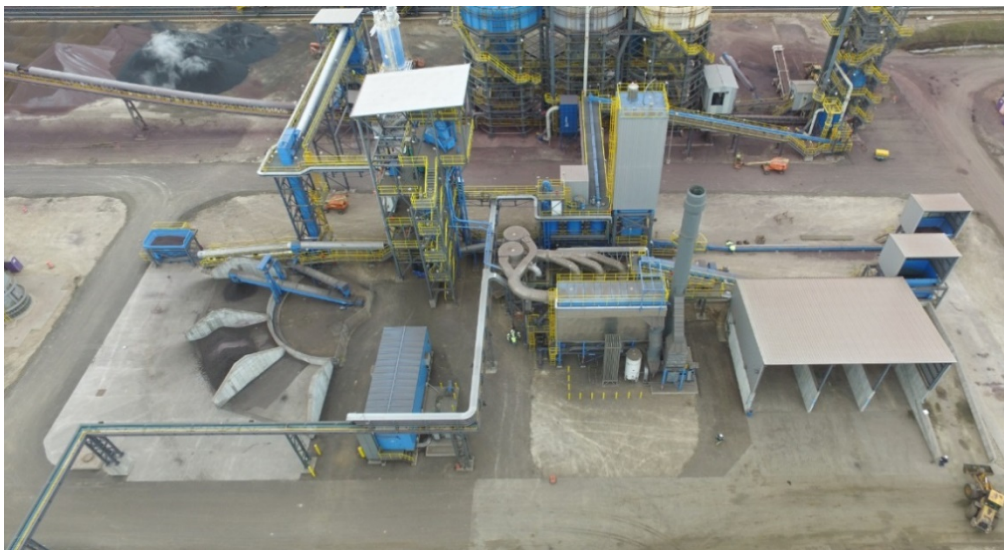
Figure 9: Picture of a cold briquetting plant for by-products as an integrated part of a DRI plant at voestalpine Texas LLC; start up 01.2017
