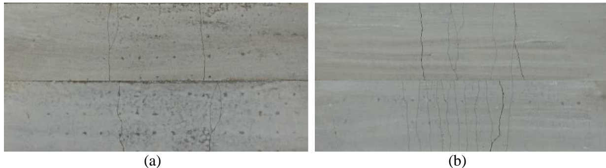
Figure 6. Typical cracking patterns for the composite: (a) R2%_50 and (b) R4%_50.
