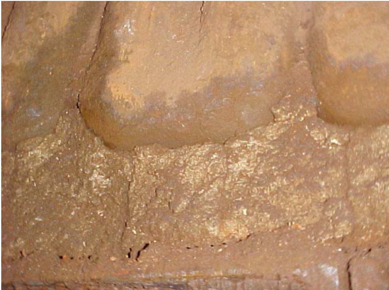
Figure 4. Severe corrosion of the cooling duct in a steel mill.
