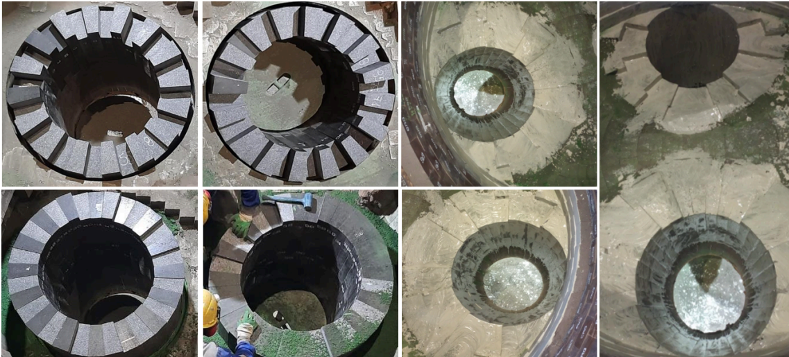
Figure 2. Refractory installation photos
