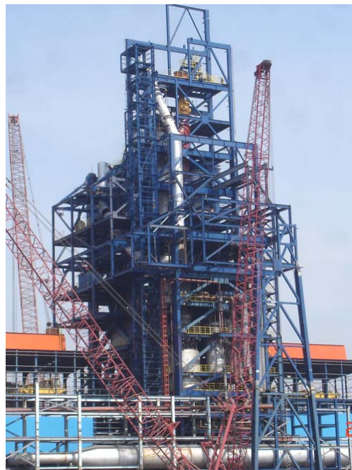
Figure 9. Construction status of COREX module 01 as of November 2007.
