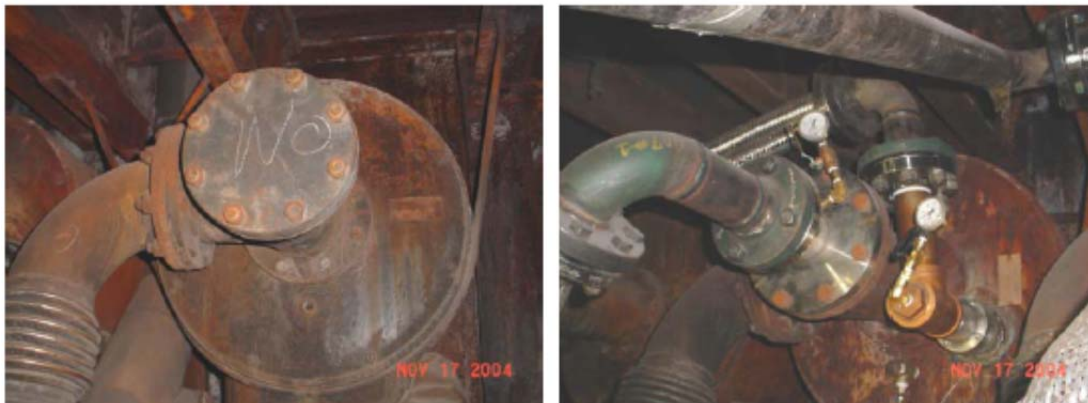
Figure 8: Reheat furnace burners (a) without DOC lances and (b) with DOC fuel and oxygen lances installed.
