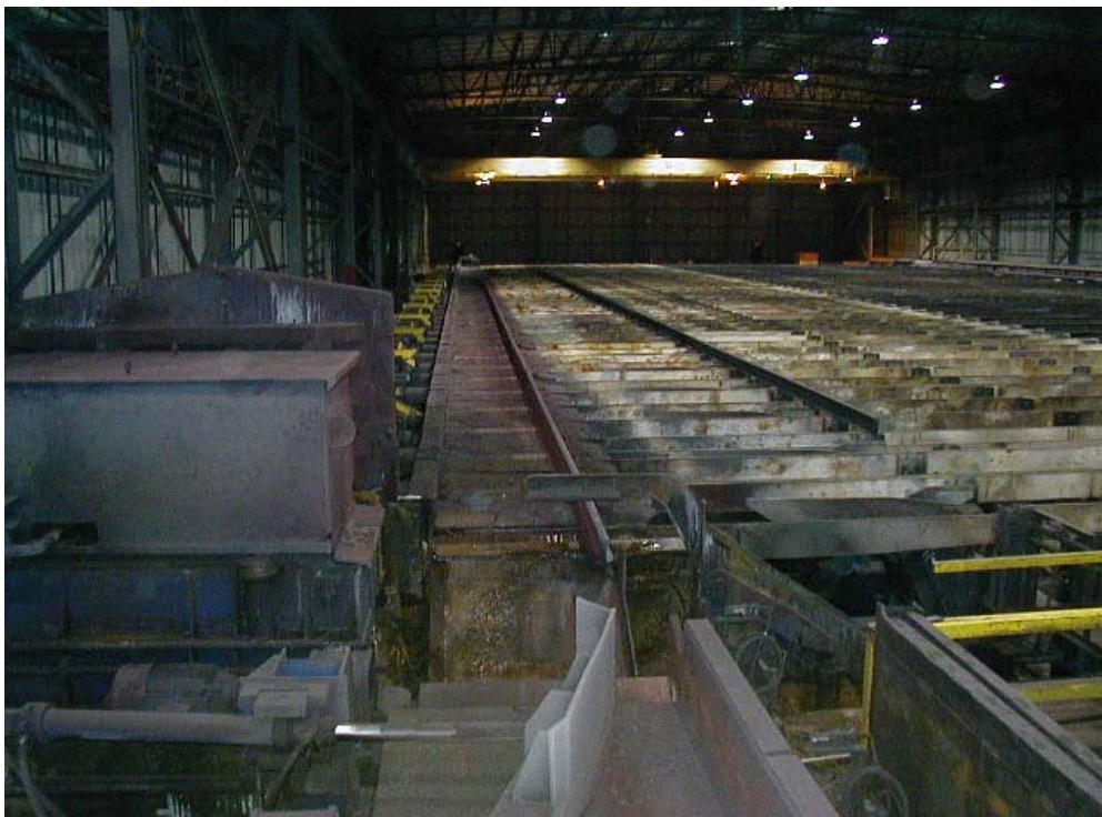
Figure 6. Cooling line for selective cooling and cooling bed.
