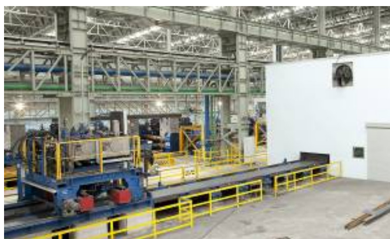
Figure 18. Cold saw with noise protection and adjustable length gauge.
