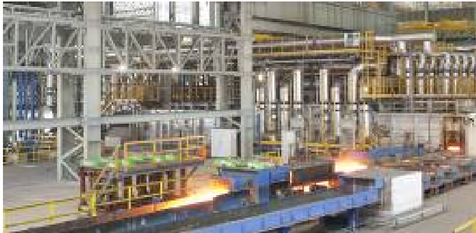
Figure 10. Ultra-low NOx reheating furnace (130 tph/160 tph).
