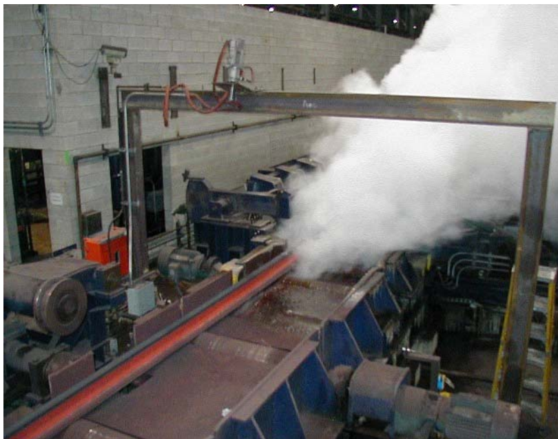
Figure 7. Cooling line for selective cooling and cooling bed.
