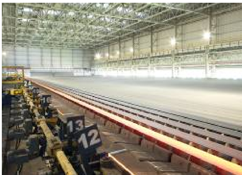
Figure 15. Quick delivery system for cooling bed.
