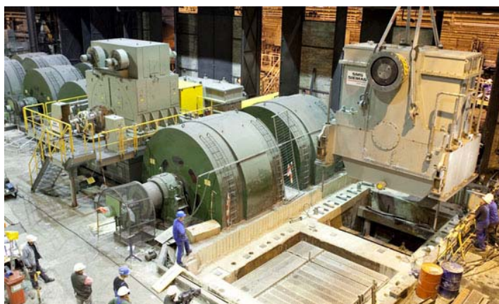
Figure 9. Insertion of finish-assembled F1 main gear unit.
