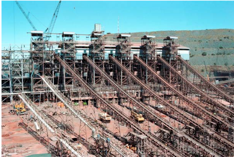
Figure 4: Iron ore jig plant, Sishen, South Africa
