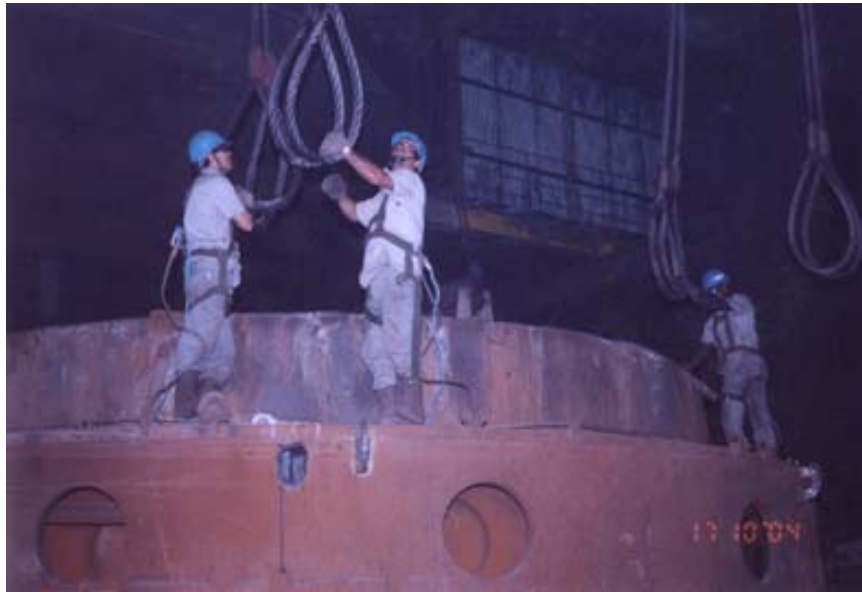
Figure 5: Dismantling of Old Converter Equipment
