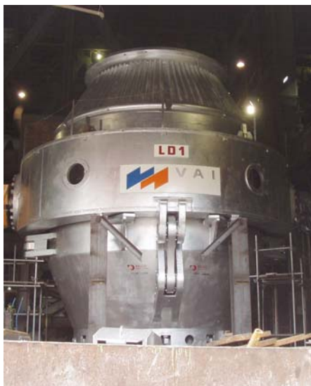
Figure 6: New Converter Equipment during Installation
