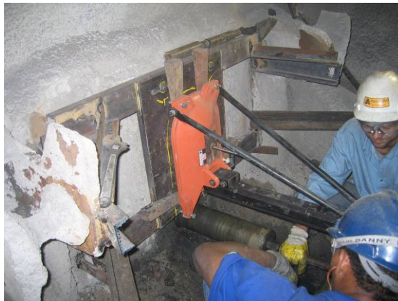
Figure 4 Drilling of hole for oxy-fuel lance
