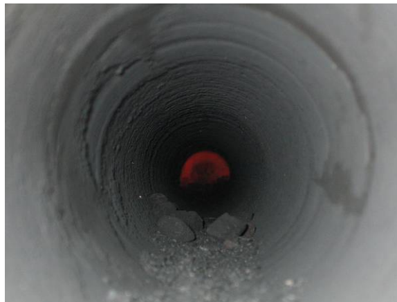
Figure 1 Severe chill: very little heat in the hearth (4.5 meter core drill through taphole)
