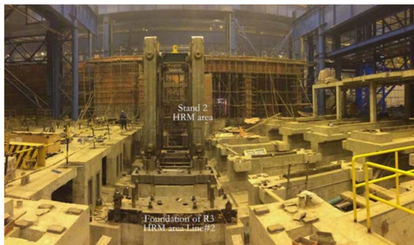
Figure 5. Line 2 under erection while Line 1 is already under commissioning.
