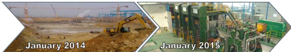
Figure 4. From ground breaking to completion within 12 months
