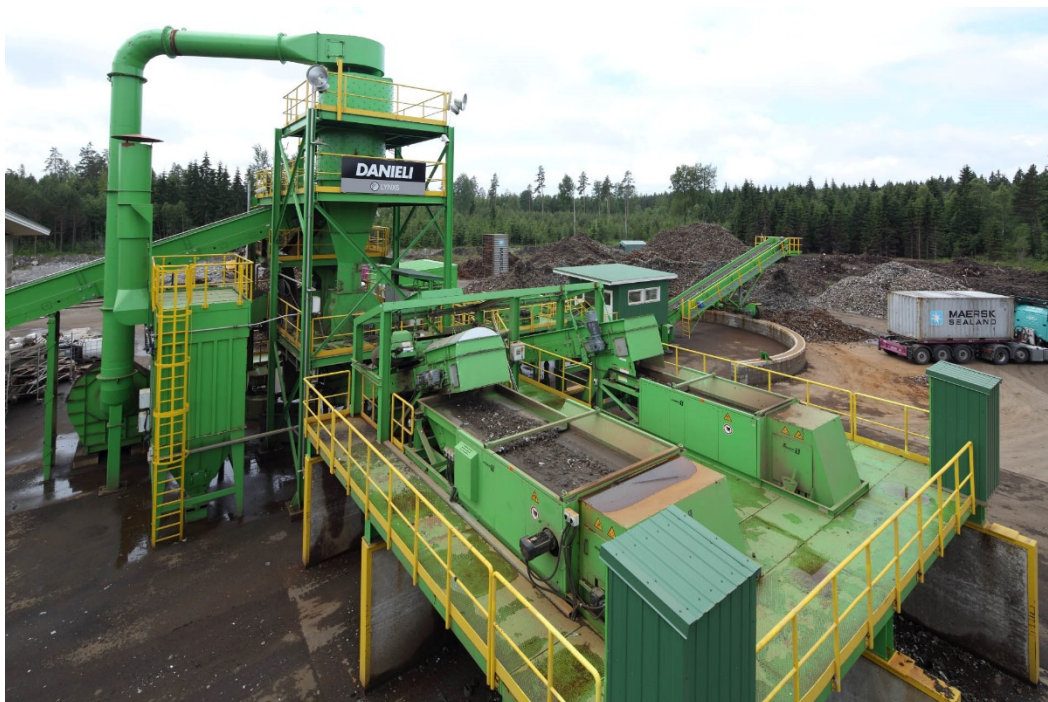
Figure 4.A recent Danieli Lynx shredder in operation
