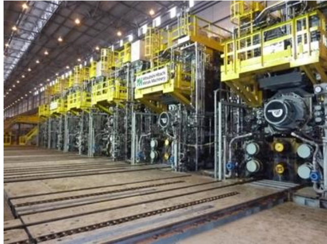
Figure 4. Finishing Mill Stands F1 to F6.
