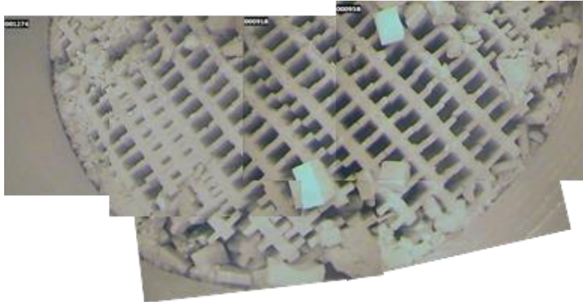
Figure 4. Endoscopic Inspection for Assessment of Stove Internals.
