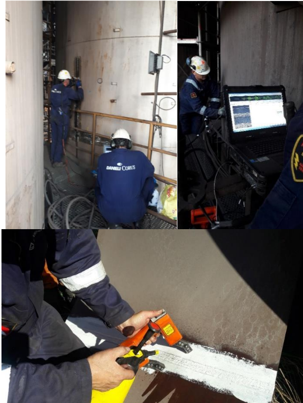
Figure 3. Shell Condition Assessment, TOFD Measurement in Progress.
