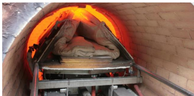
Figure 8. Burner repair while maintaining hot blast system at operating temperature.
