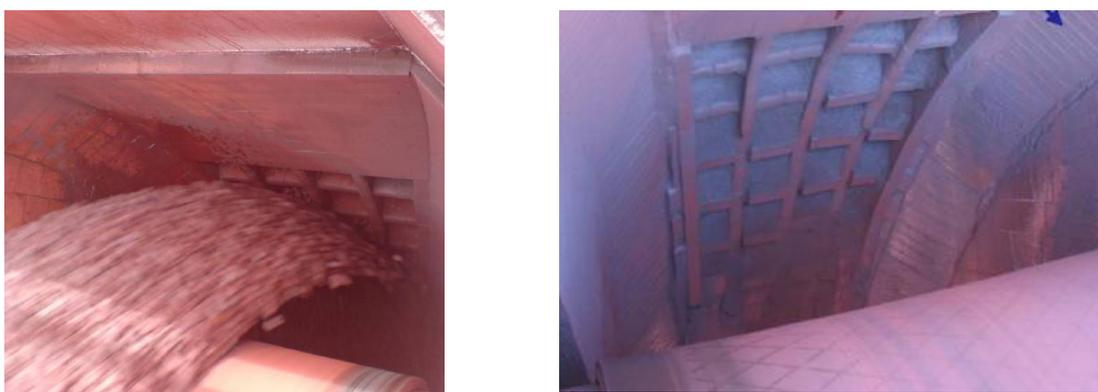
**Figure 6.** (a) Hood installation with honeycomb (b) Hood wear performance with liner plate fillet refurbishment at 3 Mt throughput
