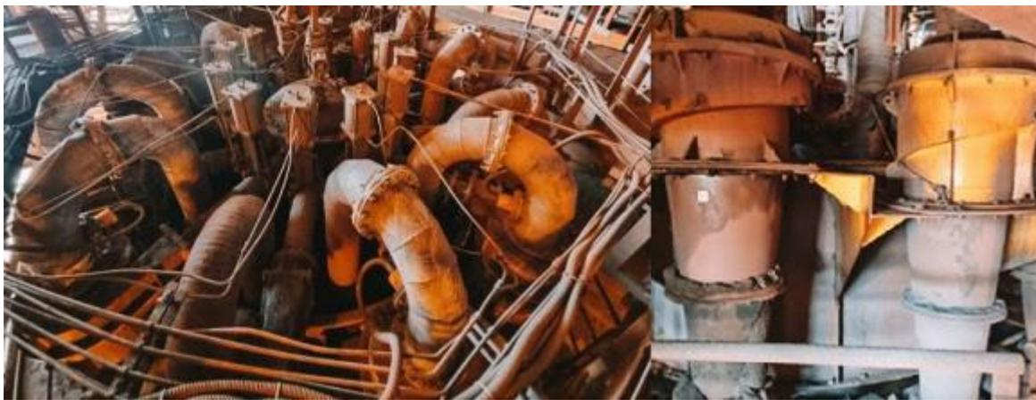
Figure 4 – Cavex® 2 CVD modules were assembled in situ.
