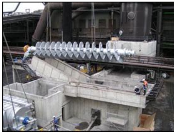
Figure 8. Installation of the Screw Conveyor.
