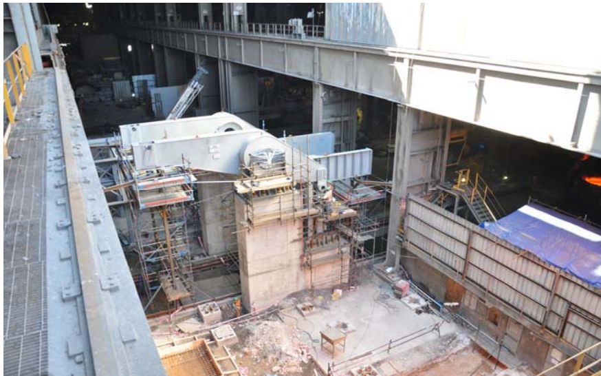
Figure 10. Rocker arms hosting sequence.
