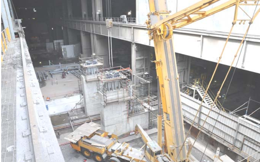
Figure 9. Foundations of the ladle rocker.
