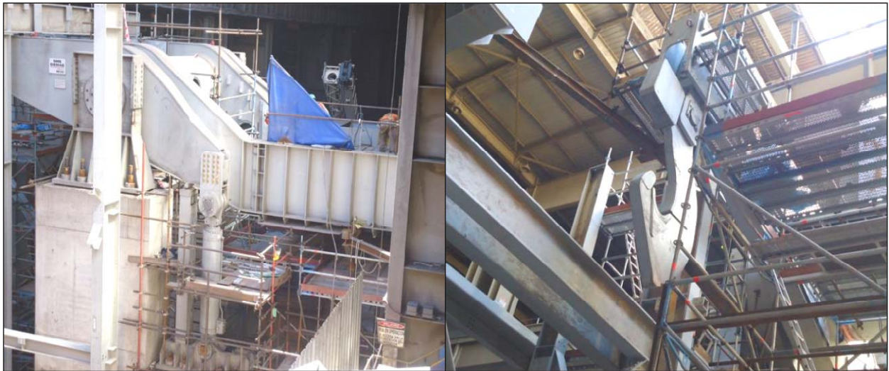
Figure 13. Hydraulic cylinder and lamella hook already placed.
