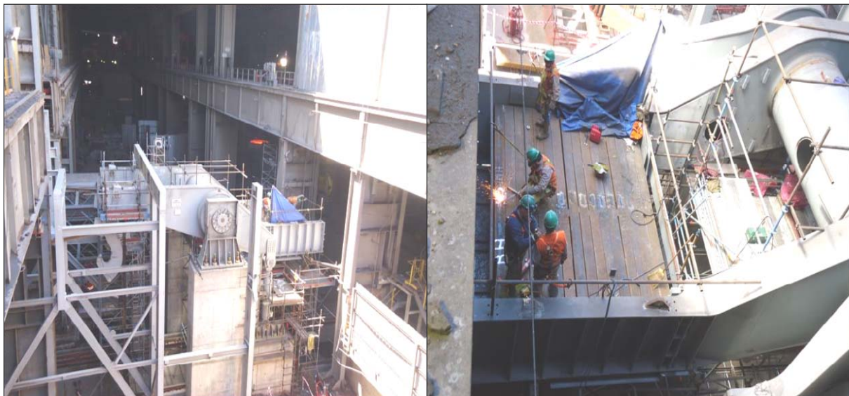
Figure 12. Fixing the counterweigh together.
