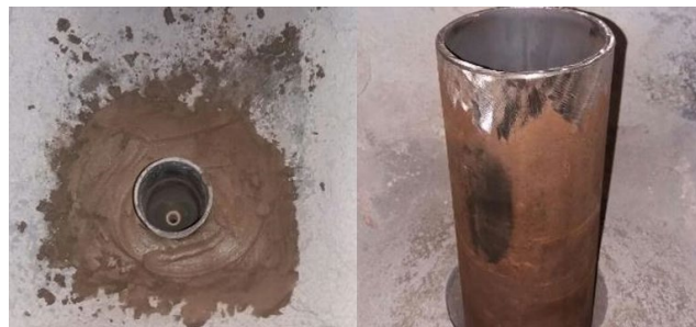
Figure 3: First starter tube, with opened top and mortar setting.
