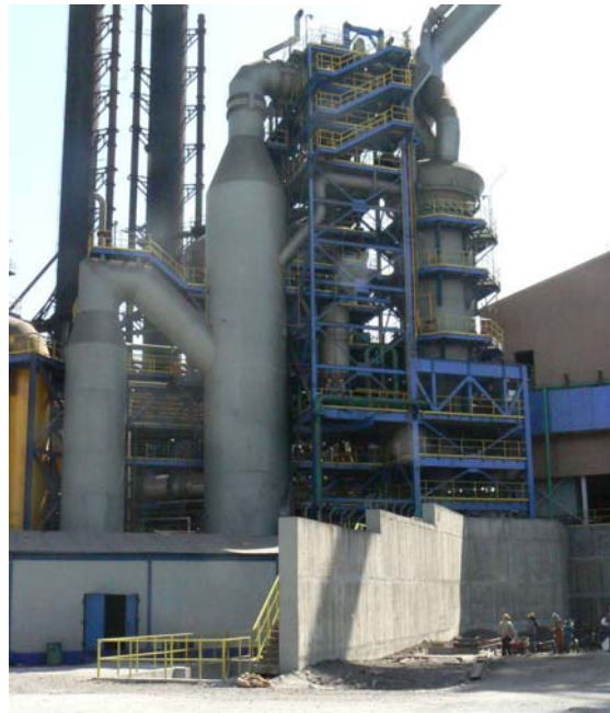
Figure 2. Gas Cleaning Plant AHMSA BF 6, 2010.
