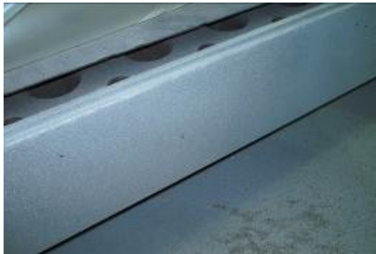
Figure 11. Broad face back-up plate after being repaired.
