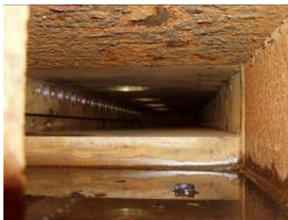
Figure 15. Inside of mold frame before blasting.
