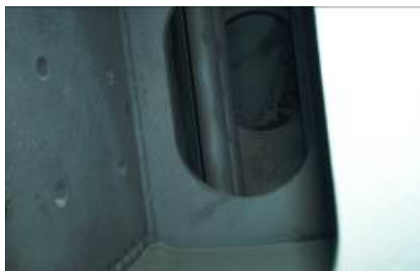
Figure 14. Interior of broad face water jacket after blasting.
