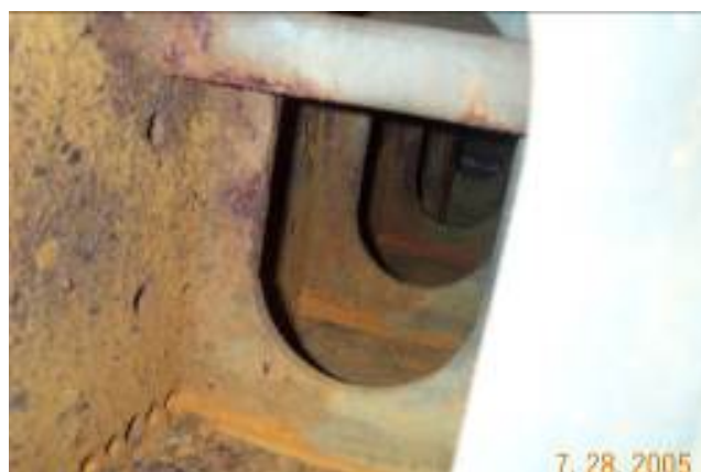
Figure 13. Interior of broad face water jacket before blasting.
