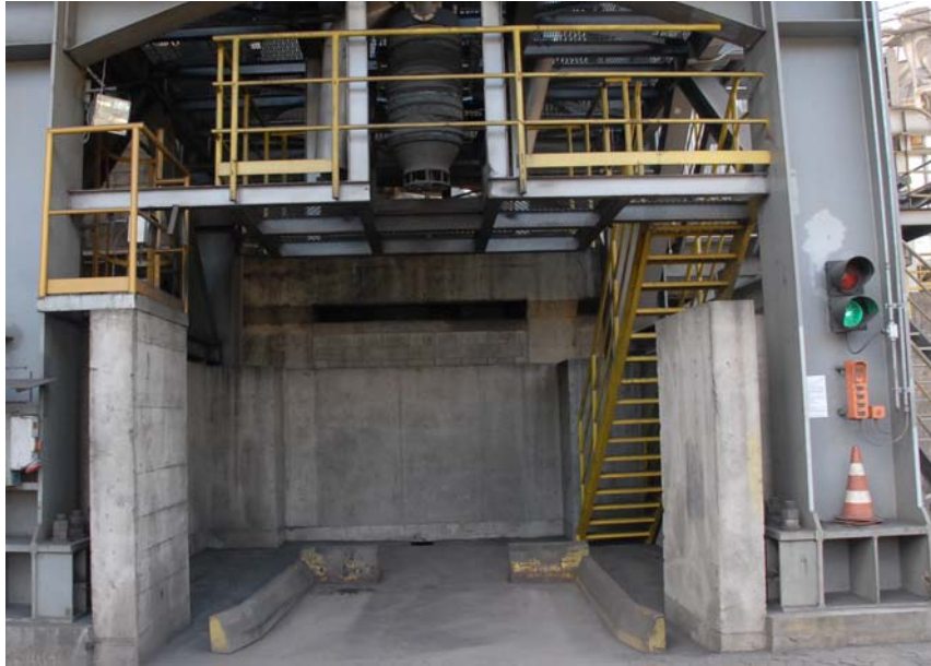
Figure 7 – Discharge area after the new BF-A gas cleaning system start-up
