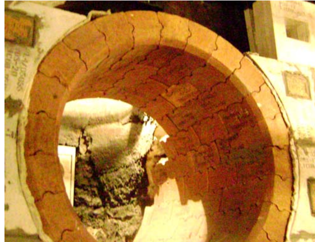
Figure 11 – New design – Lighter pieces and 3 axes fitting
