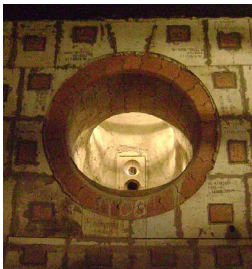
Figure 12 – Installation on chamber #8 of VALE UPSL.
