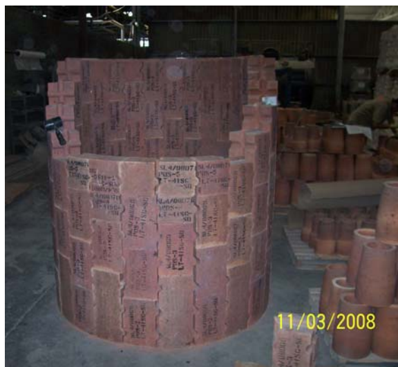
Figure 8 – Pre assembling blocks, detaches fitting and arrangement adopted.
