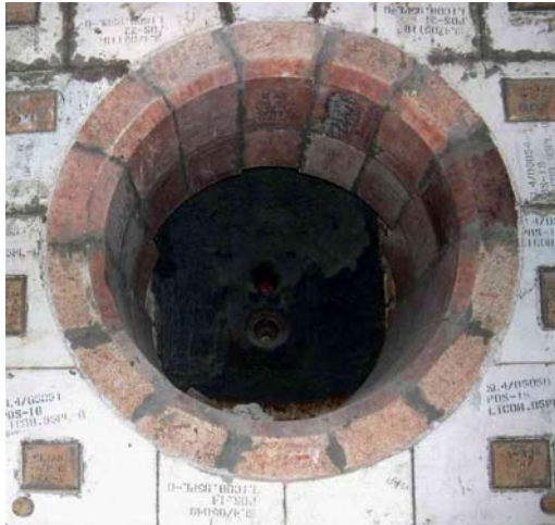
Figure 10 – “Traditional” design – detaching joint alignment
