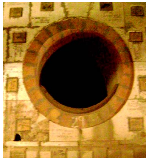
Figure 13 – Installation on chamber #29 of VALE UPSL.
