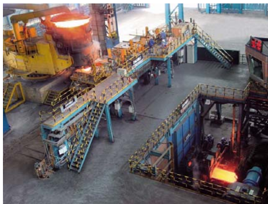
Figure 3. Overall view of the casting section at the Tangshan thin slab casting and rolling plant.
