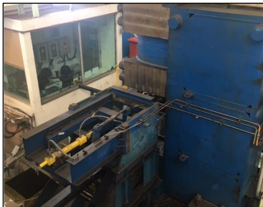
Figure 7: View of TPS and Operation Pulpit.
