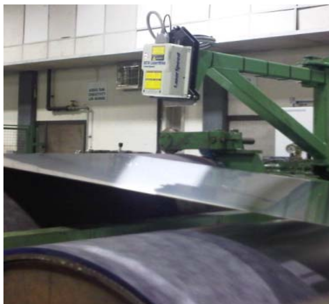
Figure 9. Tension leveler line LaserSpeed gauge installation.
