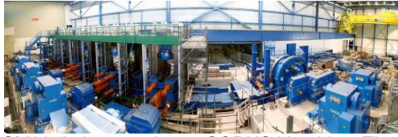
Figure 14: CM22 during erection at CORUS IJmuiden, The Netherlands
