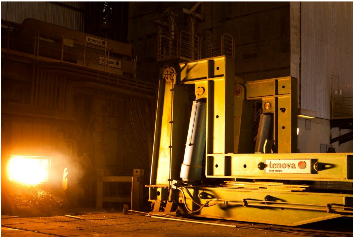
Figure 4. VSB Hot metal charging system.
