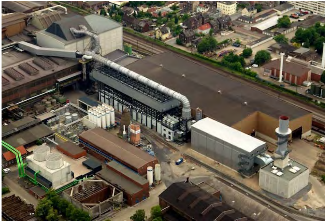
Figure 2. Dedusting plant for Peiner Träger with piping and canopy suction point.
