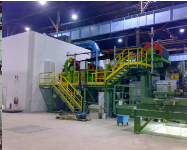
Figure 5. Steering and tension control section and the shot blasting
