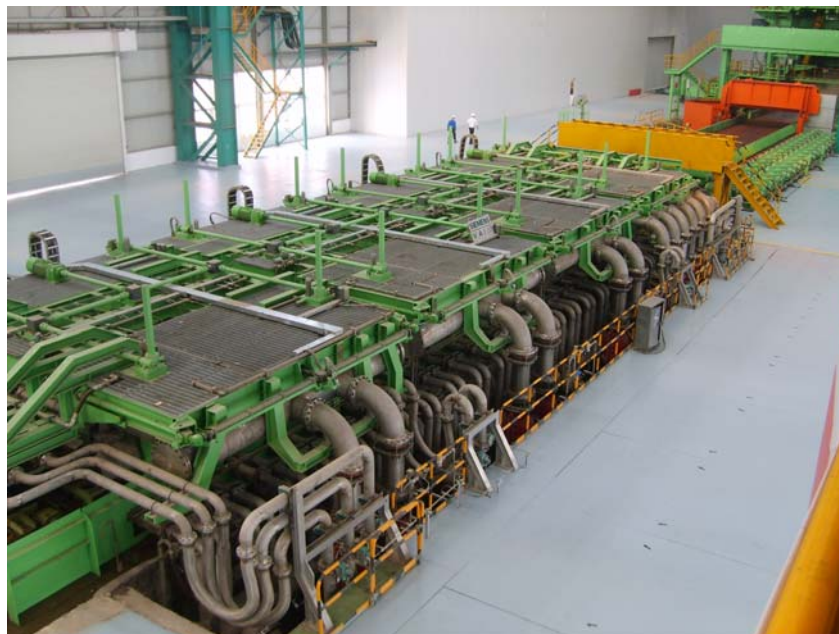
Figure 7. Mulpic line installed.
