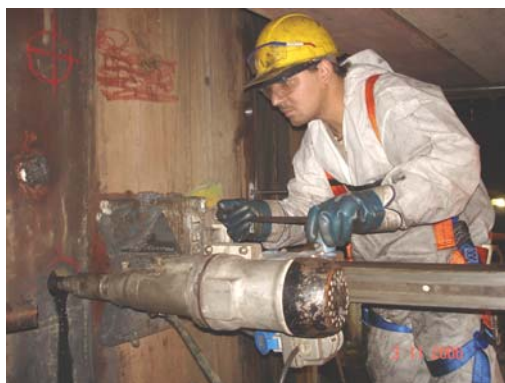
Figure 1. Equipment used to hearth core drilling.
