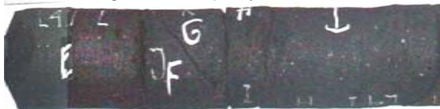
Figure 5. Cracked carbon: 500 mm.
