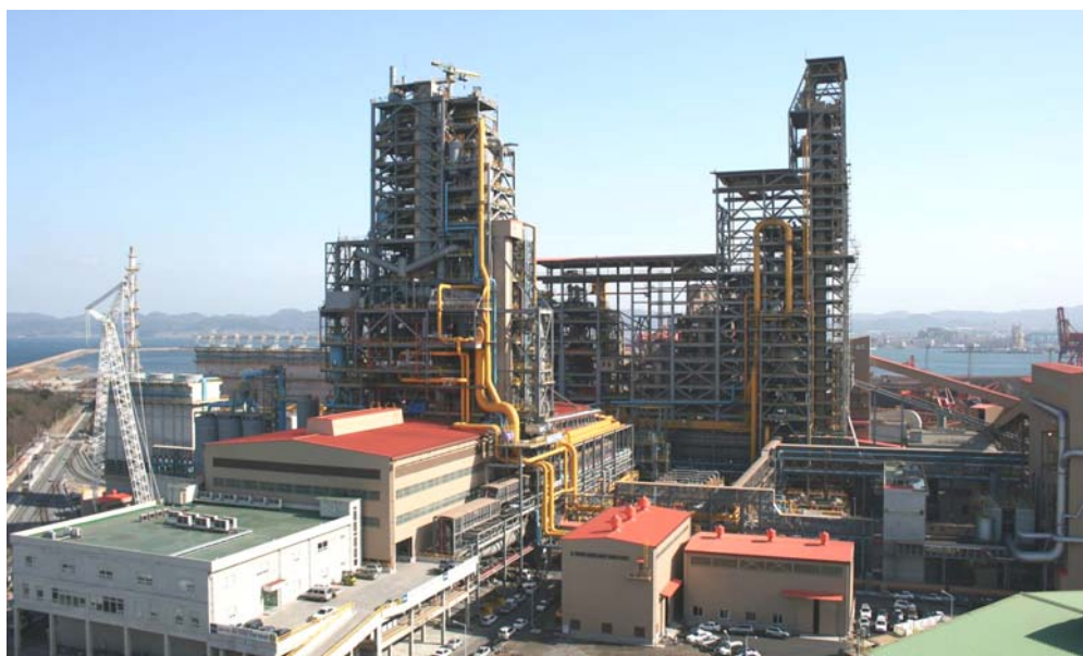
Figure 3 FINEX ® 1.5 Mt/year Plant
