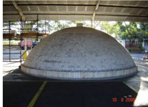
b) Pre-Assembly of Dome Roof.
