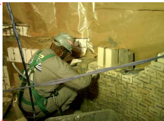
c) Combustion Chamber Assembly
