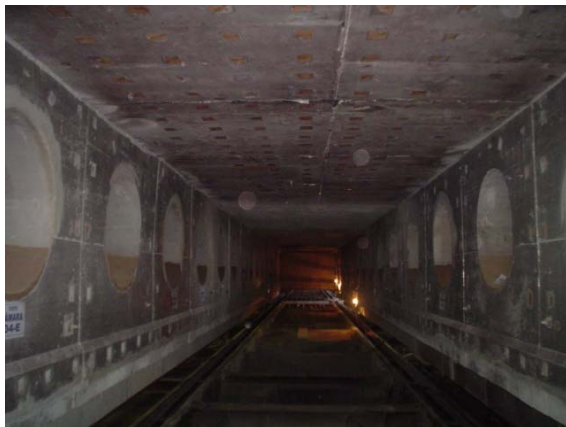
Figure 10 – Furnace with monolithic lining
