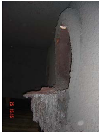
Figure 3 - Formation of "scab" in combustion chambers
