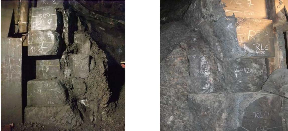
**Figure 2.** Hearth walls with brittle layer.
