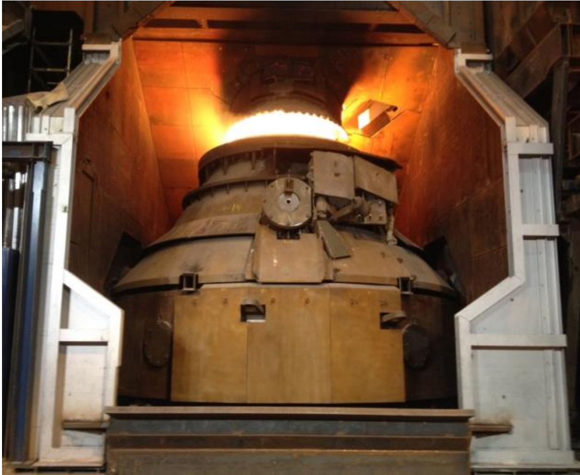
Figure 4 : LD (BOF) converter supplied by Primetals Technologies at the Finnish Raahen works of SSAB Europe Oy.
