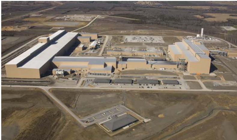
Figure 2: SeverCorr plant with cold mill complex, CSP ® plant and steelmaking plant (from left to right).
