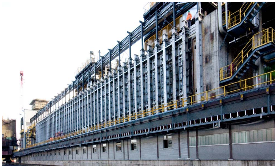
Figure 1. New coke oven Battery N° 3 of ZKS.
