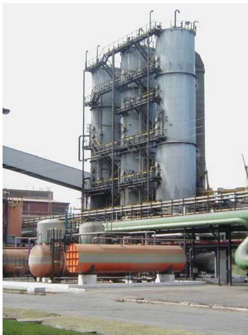
Figure 9. Gas scrubbers for 100000 Nm 3 /h to remove NH 3 , H 2 S, C 10 H 8 .
