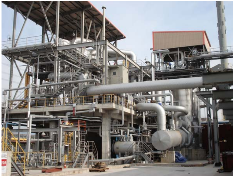
Figure 11. A claus plant for high purity sulphur recovery
