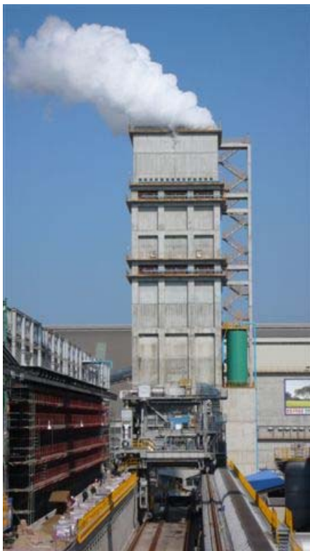
Figure 2. CSQ quench towers at Hyundai and Schwelgern coke plant.
