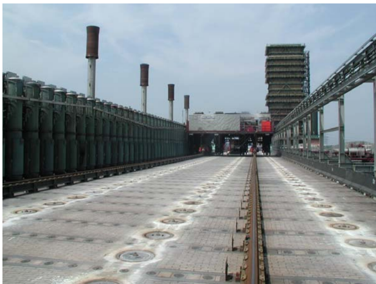
Figure 8. The Schweglern battery in operation - emission free thanks to PROven.™
