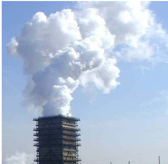
Figure 2. CSQ quench towers at Hyundai and Schwelgern coke plant.
