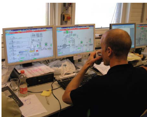
Figure 5. Hlsarna control room
