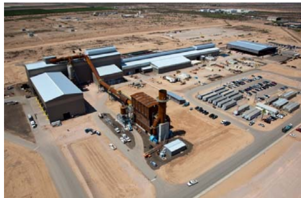
Figure 19. Site prior to commissioning
