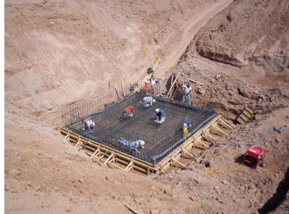
Figure 17. First concrete pour, late 2008
