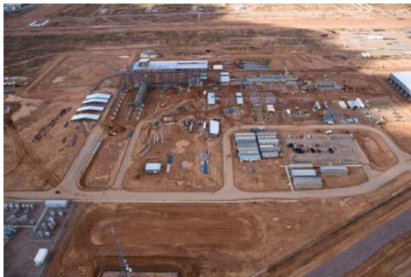
Figure 18. Site midpoint thru construction
