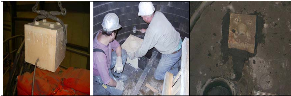
Figure 4- Installation of CSB in ladle bottom.
