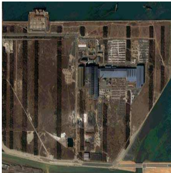
Figure 1: Job site for Dragon Steel integrated steel works.
