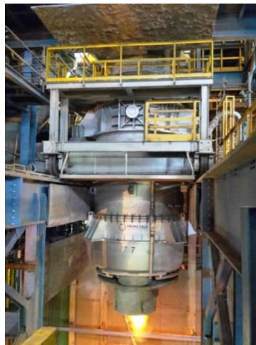
Figure 3 RH vessel including vessel transfer car
