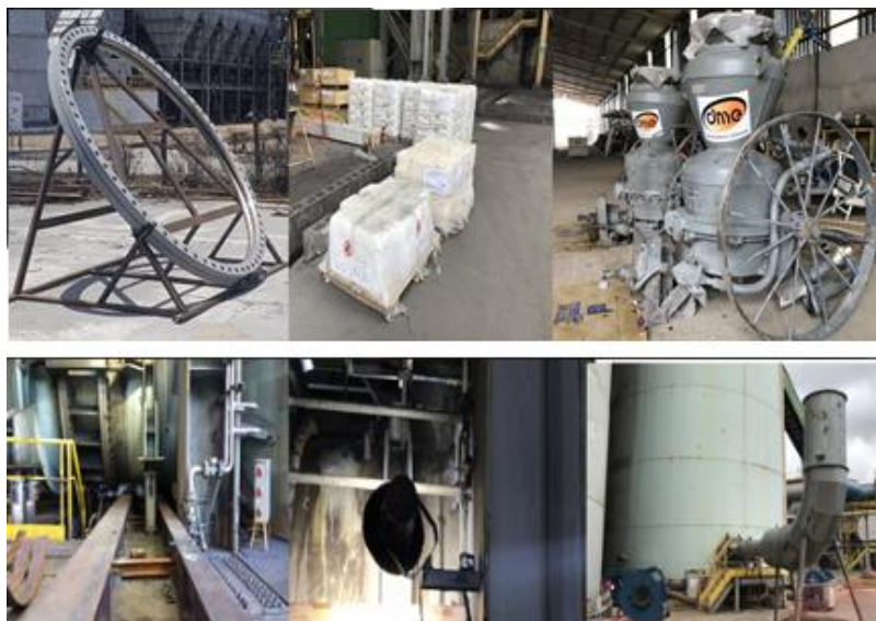
Figure 14. Full Services: Engineering, Fabrication, Equipment development, wire cutting under hot conditions, Heating up and thermal comfort, eletromechanical and refractory activities
