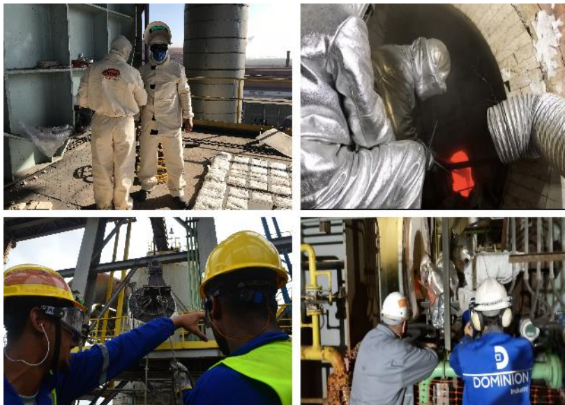
Figure 12. Repair Team on site activities
